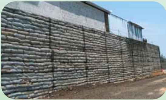
Commercial Center Parking Lot Project in Jalapa, Ver., Mexico
