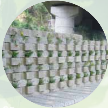
Modular block reinforced structure
