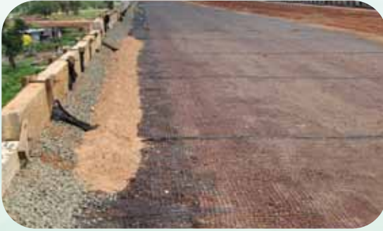
Highway Construction Project in Shivpuri, India
