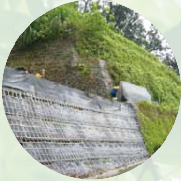
Steel mesh reinforced structure
