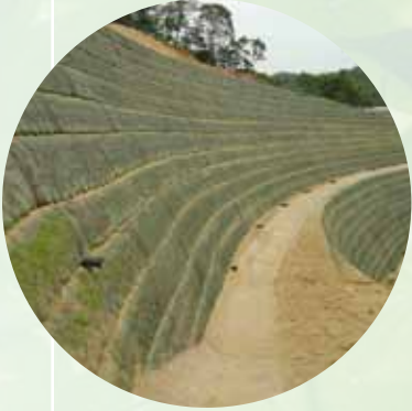
Wrap-around reinforced structure
