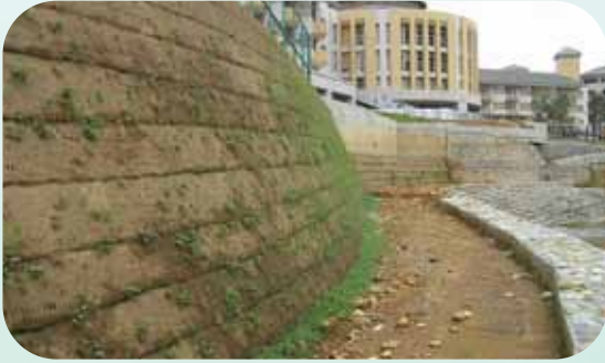
Athletic Field Landscape Construction in Pu-Tai Elementary School Project
