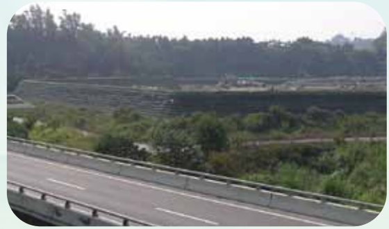
Jhuci Landfill Construction Project in Chia Yi
