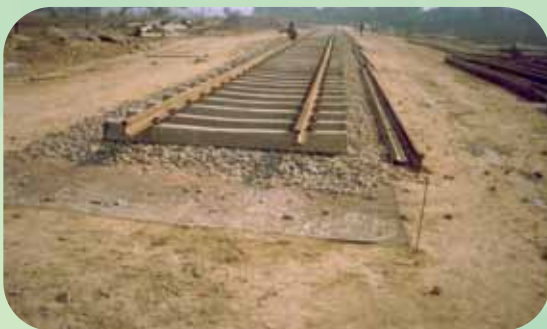
Railway Foundation Reinforcement in India
