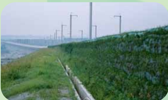
Crash Barrier Embankment in Taiwan HSR C250 Project
