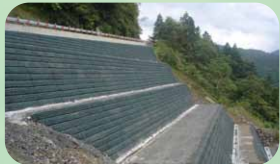
Yilan First Road Roadbed Repair Construction Project
