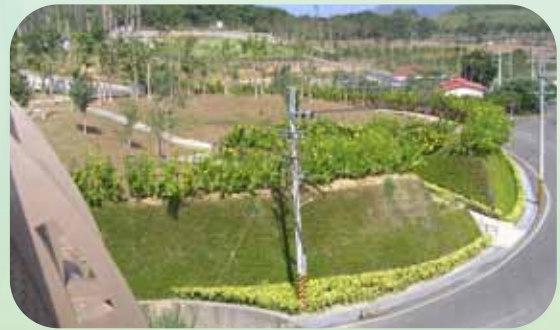
Conservation Zone Construction Project in Pu-Tai Elementary School
