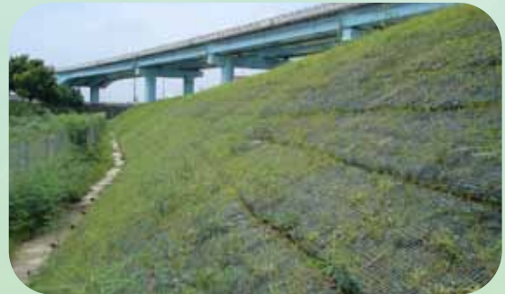
Taipei Rapid Transit Metro System Tucheng Line Depot Construction
