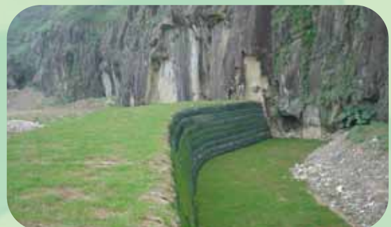
Rockfall Barrier Embankment in Badouzhi, Keelung
