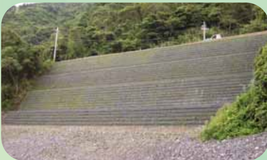
Nantou No.83 Road Repair Construction Project
