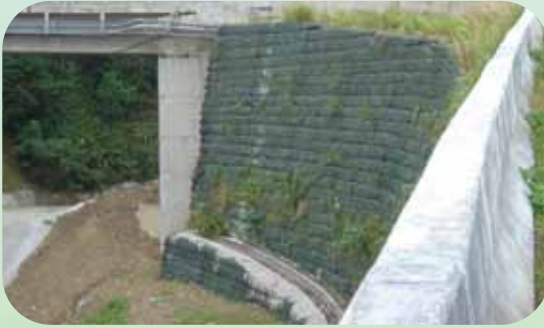
Abutment Construction in Tamkang University Lanyang Campus
