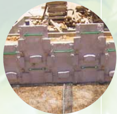
Precast concrete panel reinforced structure
