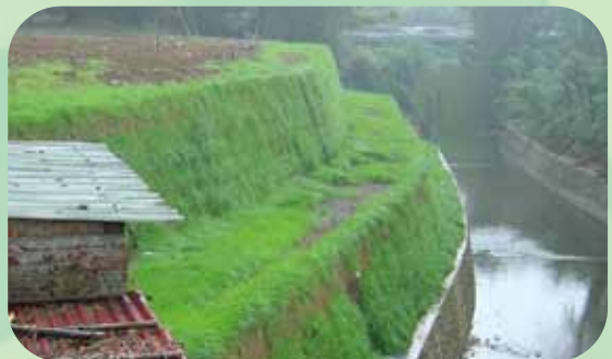
Reinforced Structure Construction Project near the Channel in Tao Yuan
