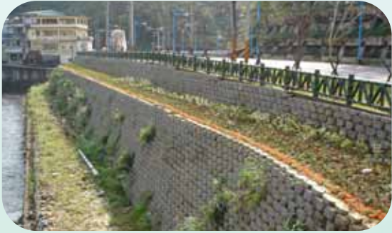
Shuangsi No.1 Road Construction Project in Shuangsi River Section
