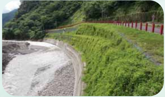
Nantou No.80 Road Repair Project in Beikang River Section
