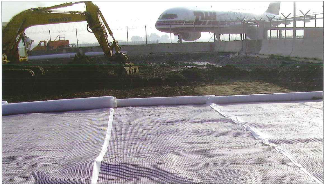
Pisa airport, Italy - Ground stabilisation with TENAX GT geocomposite
