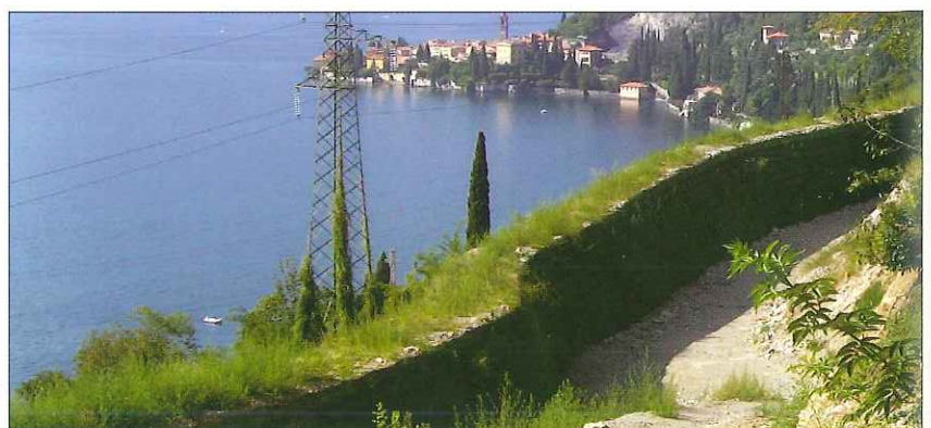
Lake of Como, Italy - Rockfall barriers to protection the historical village of Varenna
