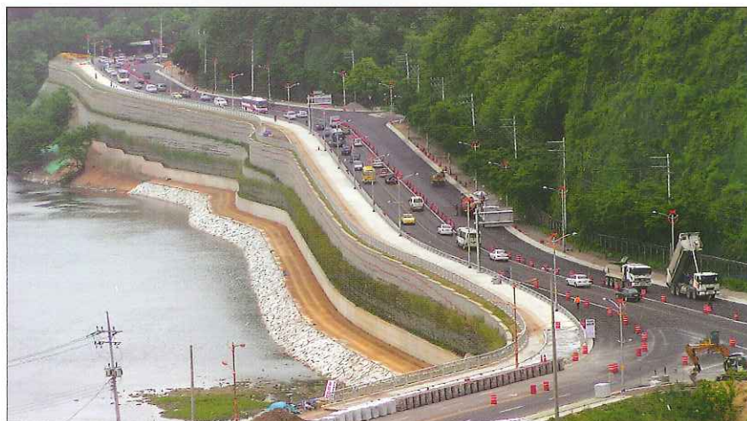
South Korea, Chunsugyo Saebeari Highway - Geoblock segmental retaining wall System.
