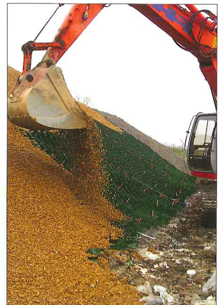
Modena landfill , Italy - Construction of embankment alongside high-speed railway line.
