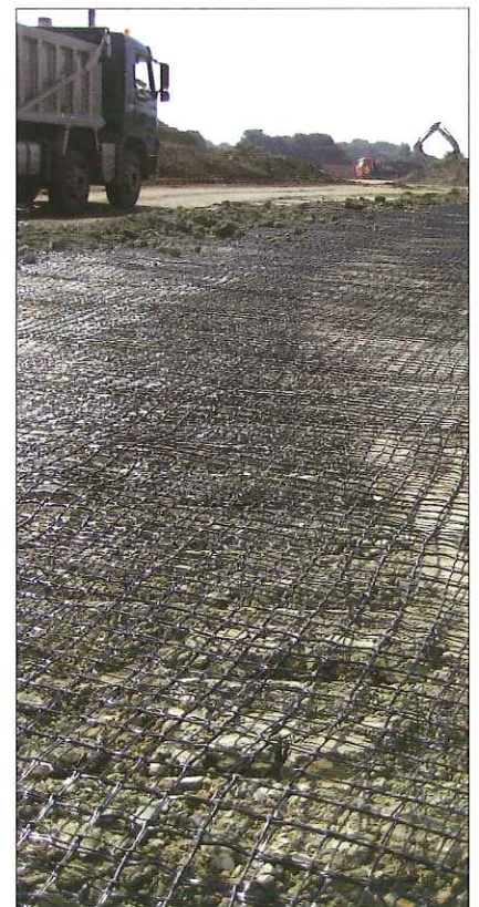
Abraham Darby Academy, Telford, UK - Control of differential settlements using 3D Grids
