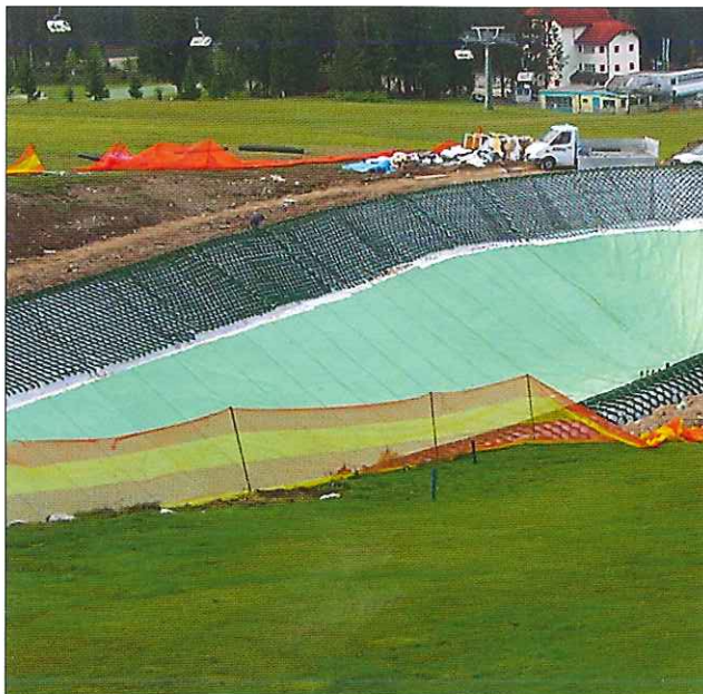
Below: Carezza Lake, Italy - Facing of the walls to protect the PVC waterproofing.
