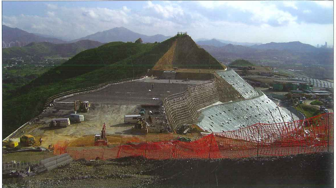
35m high reinforced soil embankment constructed to retain future waste fill in NENT landfill, Hong Kong.
